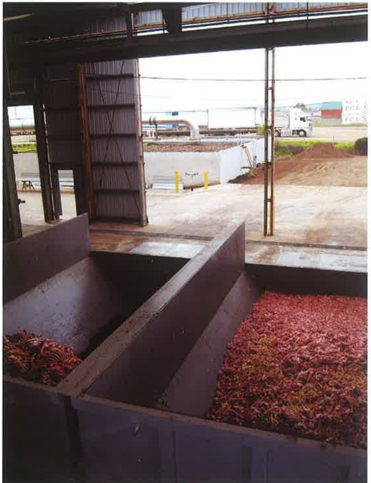
The new raw material holding bins allow separation of materials. The biofilter extension can be seen in the background.
